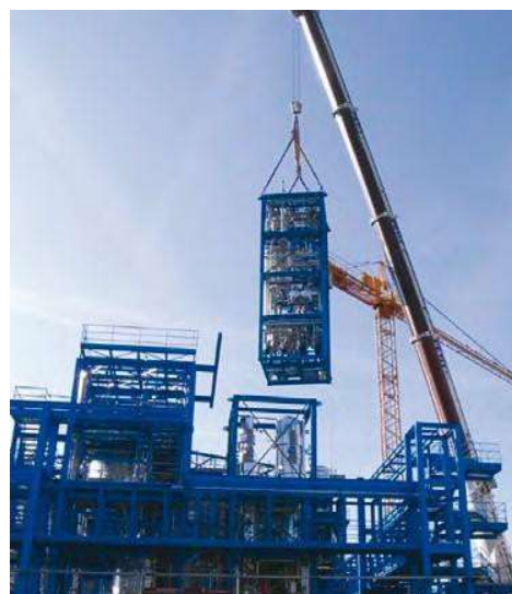
INSTALLATION OF DOUBLE STAGE SKID-MOUNTED EVAPORATOR FOR AGROCHEMICAL CONCENTRATION
